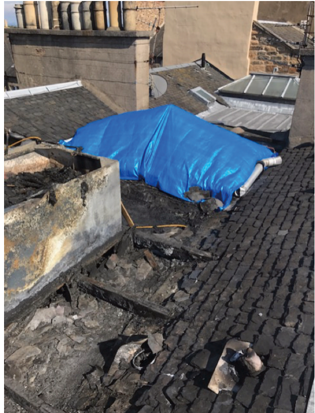
Image 2. Fire damage to the roof
