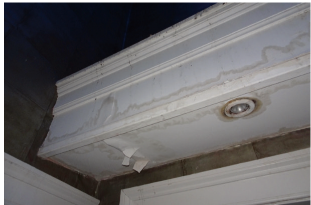
Image 3. Internal water damage to bespoke fixtures and fittings
